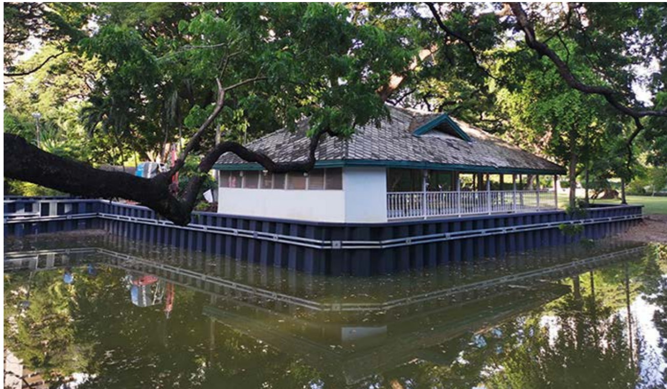
BANGKOK, THAILAND: VINYL SHEET PILES USED TO DEVELOP BLUE INFRASTRUCTURE AT THE US EMBASSY.
