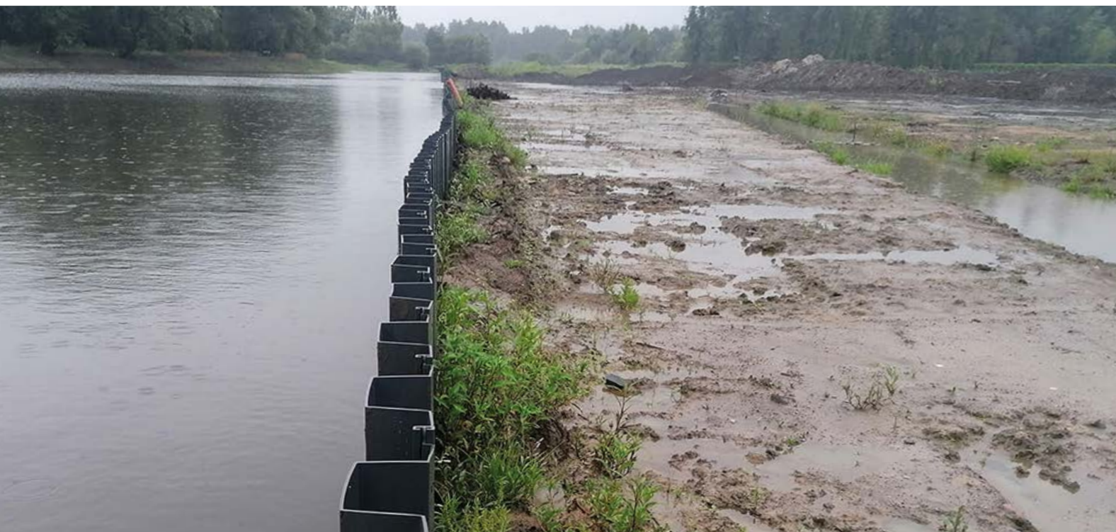
KOMORÓW, POLAND: VINYL SHEET PILES WITH GASKETS USED TO TEMPORARY REDIRECT THE RIVER BED.
