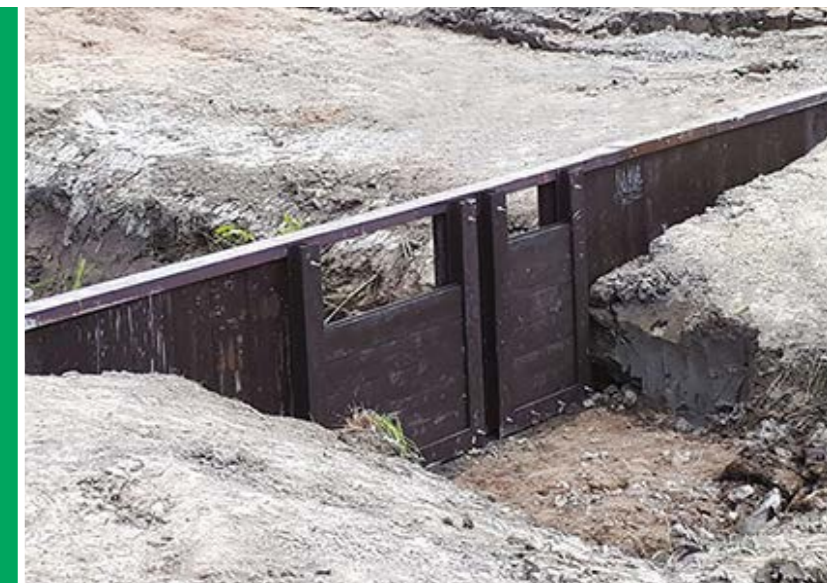
SWEDEN: FIRST VINYL SMALL RETENTION SLUICE INSTALLED OUTSIDE POLAND.
