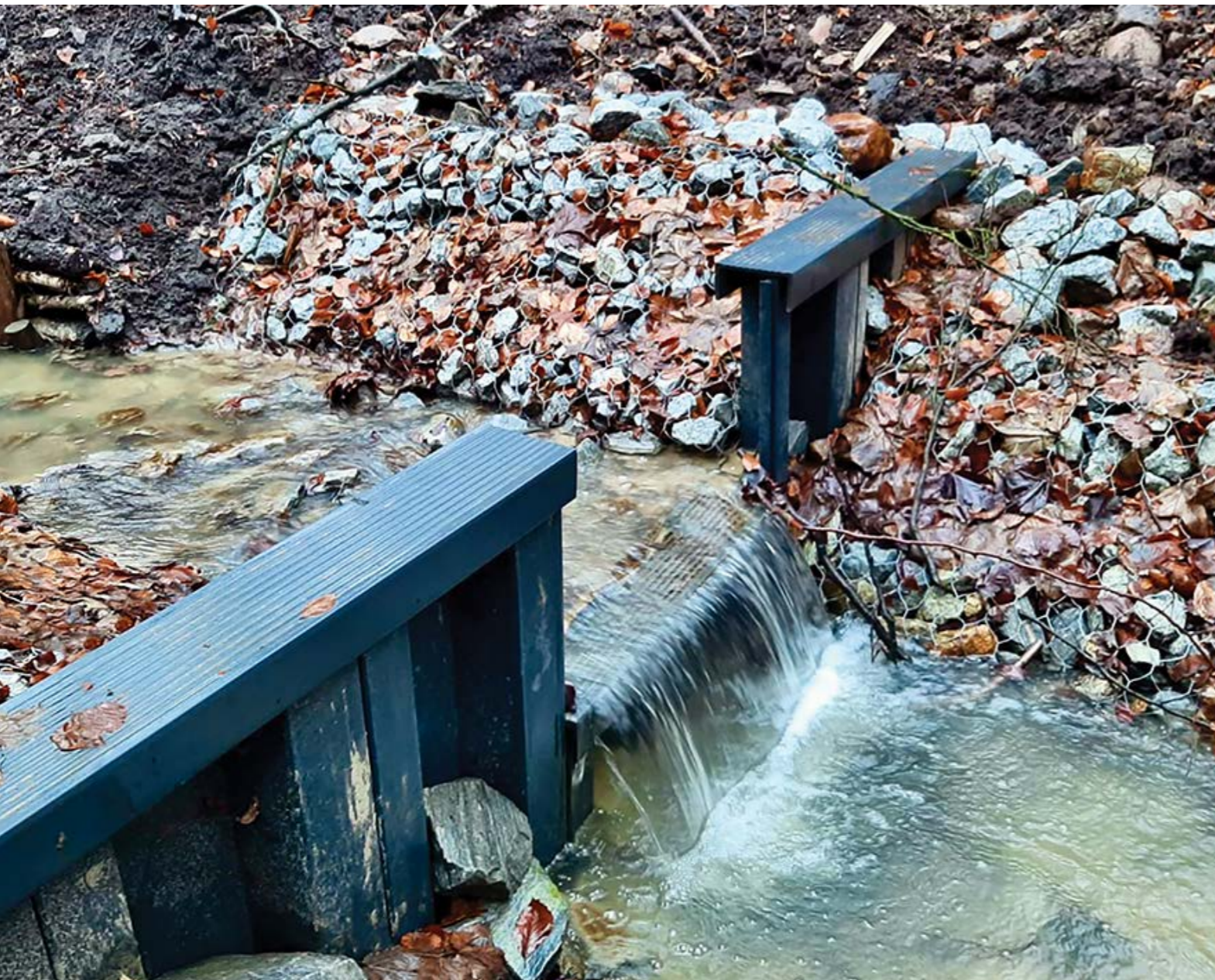
SZCZECIN, POLAND: SYSTEM OF WATER BARS INSTALLED AT A STREAM TO SLOW DOWN WATER RUN-OFF.
