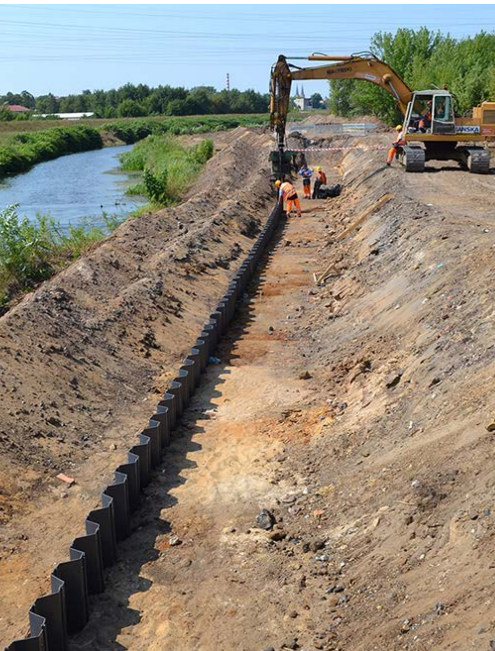
CZĘSTOCHOWA, POLAND: REINFORCEMENT OF A FLOOD EMBANKMENT.
