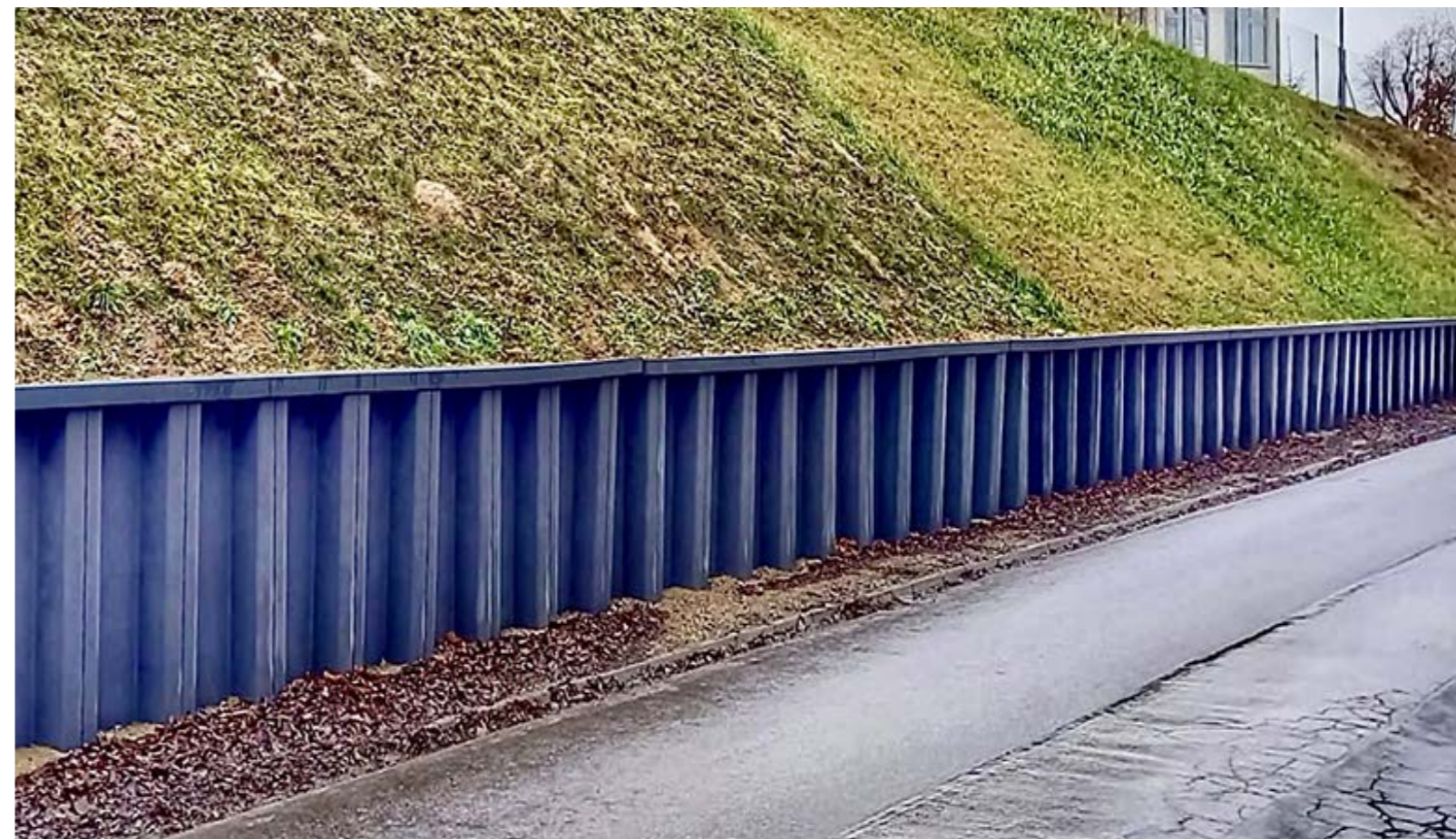
THE CRACOW AREA, POLAND: STABILIZATION OF A STATE ROAD EMBANKMENT.
