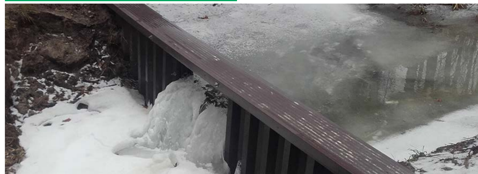
THE PODANIN FOREST DISTRICT, POLAND: VINYL SMALL RETENTION SLUICES ARE DURABLE AND RESISTANT TO ATMOSPHERIC CONDITIONS.
