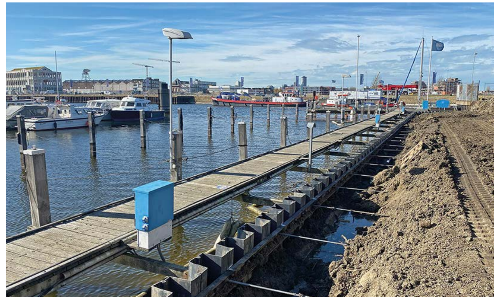
VLISSINGEN, THE NETHERLANDS: VINYL SHEET PILING WALL REINFORCED WITH EARTH ANCHORS IN A HARBOUR DEVELOPMENT PROJECT.
