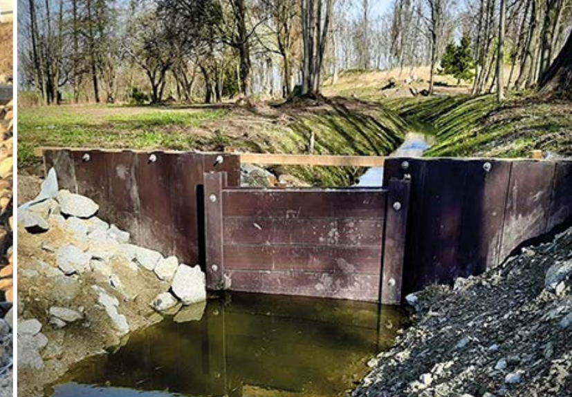
THE JAROCIN AREA, POLAND: SMALL RETENTION SLUICES INSTALLED IN A DEVELOPMENT PROJECT OF A MUNICIPAL PARK.
