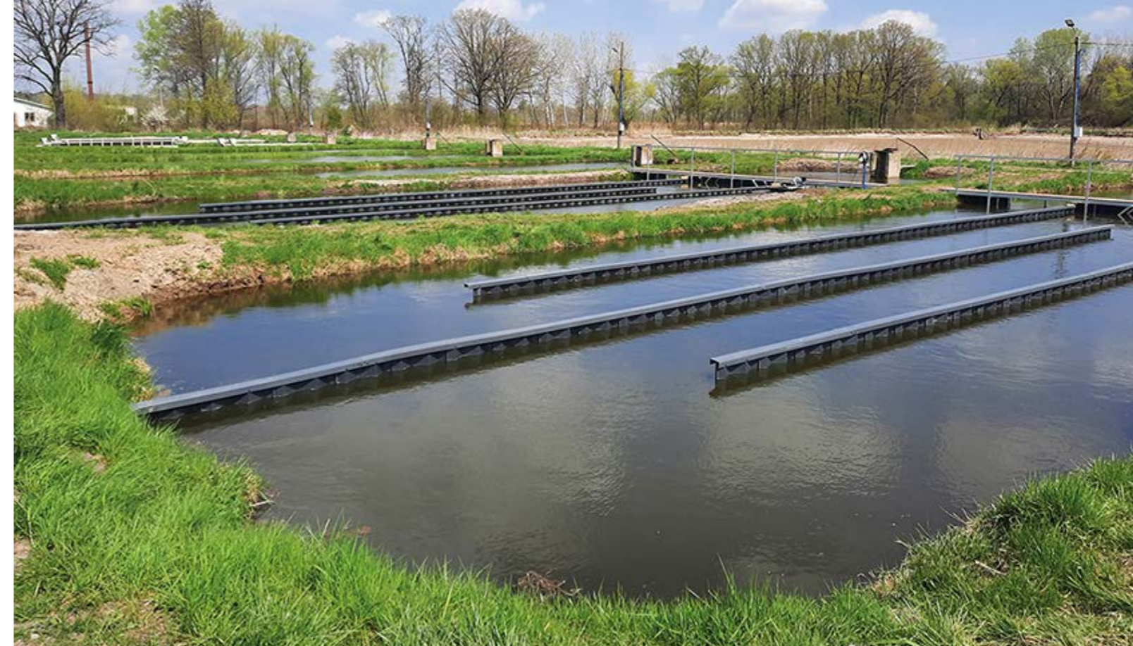
VINYL SHEET PILING AND TERRADECK COMPOSITE PLANKS USED TO CONSTRUCT THE INFRASTRUCTURE OF EXPERIMENTAL FISHING PONDS IN ŻABIENIEC, POLAND.
