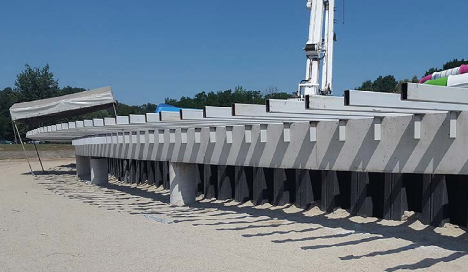
NYSA, POLAND: VINYL SHEET PILING USED TO CONSTRUCT A MUNICIPAL WATER PARK.
