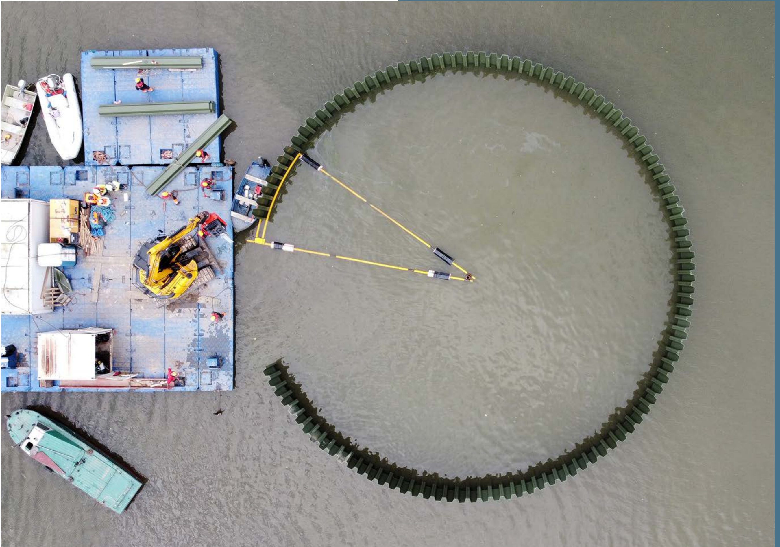
THE GOCZAŁKOWICE LAKE, POLAND: CONSTRUCTION OF AN ARTIFICIAL BIRD ISLAND.
