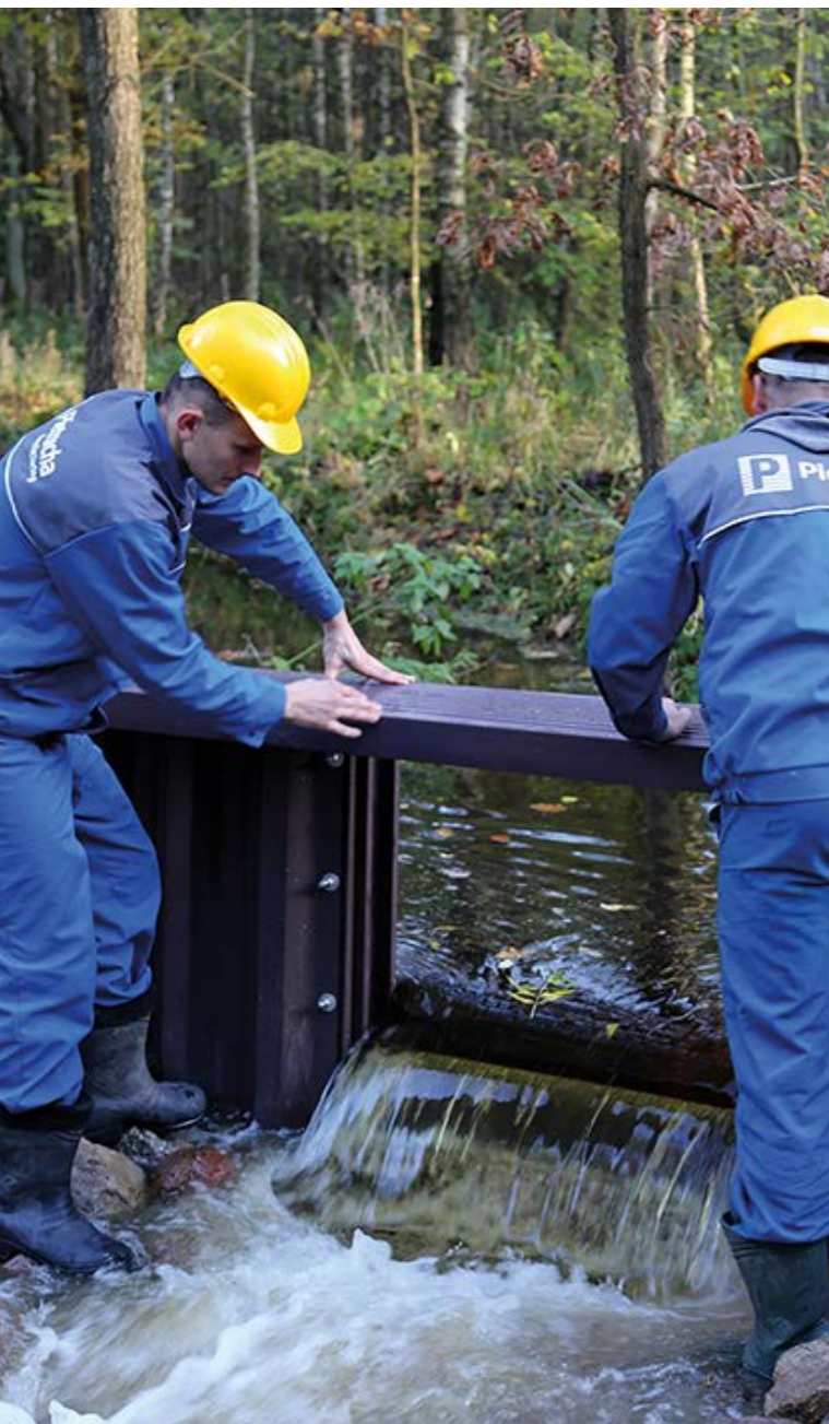
THE POZNAŃ VOIVODESHIP, POLAND: INSTALLATION OF A VINYL SMALL RETENTION SLUICE TO PROTECT A FOREST ECOSYSTEM AGAINST DROUGHTS.
