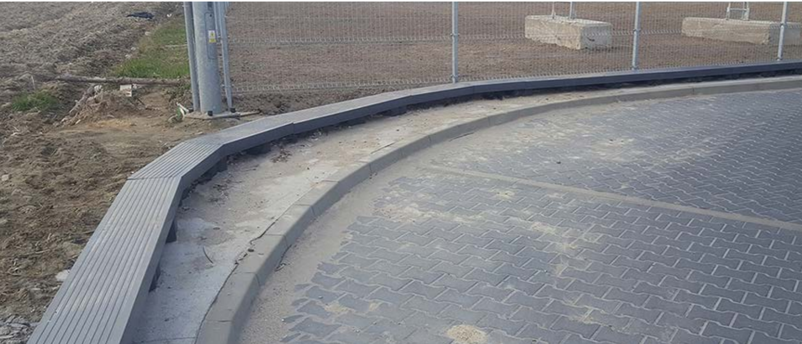
KUTNO, POLAND: PROTECTION OF A PETROL STATION AGAINST FLOODING FROM THE SURROUNDING FIELDS, ENHANCING THE RETENTION CAPACITY OF THE AGRICULTURAL AREA BY REDIRECTING THE WATER FILTRATION ROUTE, AS WELL AS PROTECTING THE ADJACENT FARMING LAND AGAINST POSSIBLE CONTAMINATION WITH CHEMICAL SUBSTANCES.
