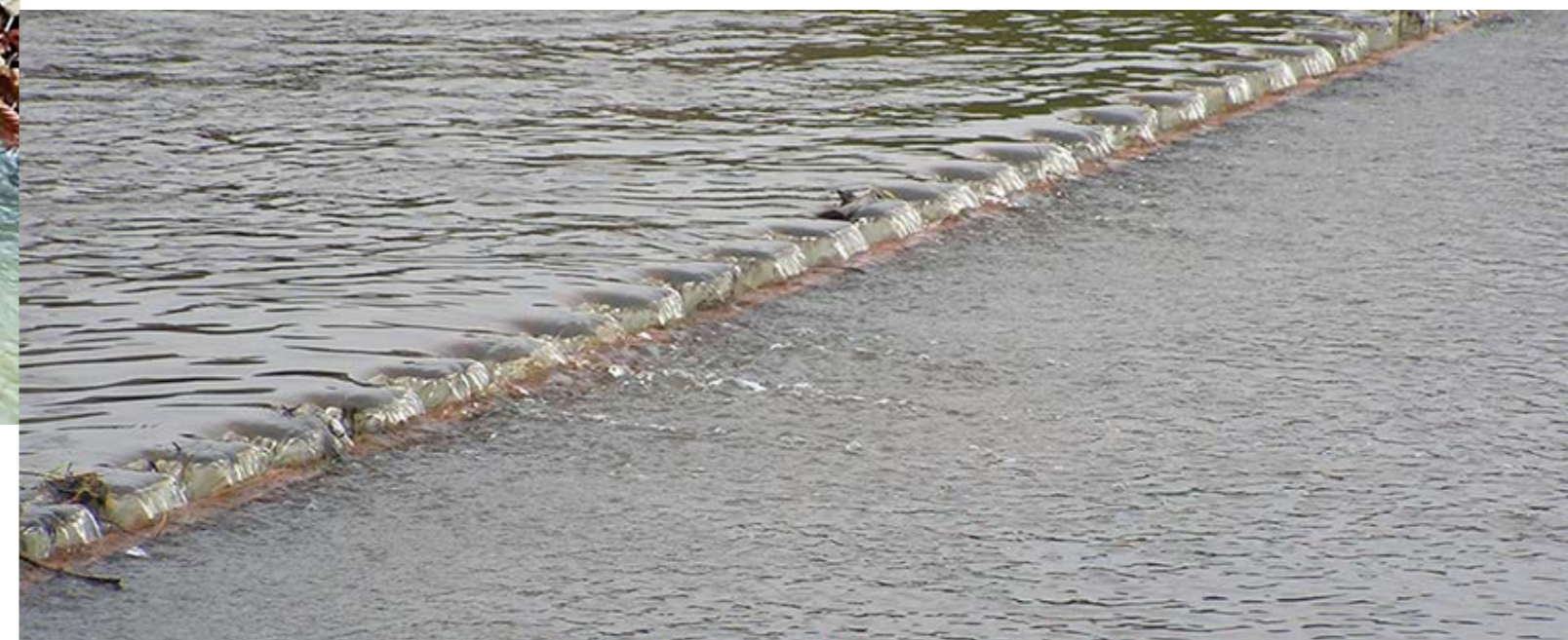
BIESTRZYNNIK, POLAND: ECOLOCK VINYL SHEET PILES USED TO CONSTRUCT A WATER BAR ON THE LIBAWA RIVER IN THE ODER BASIN.
