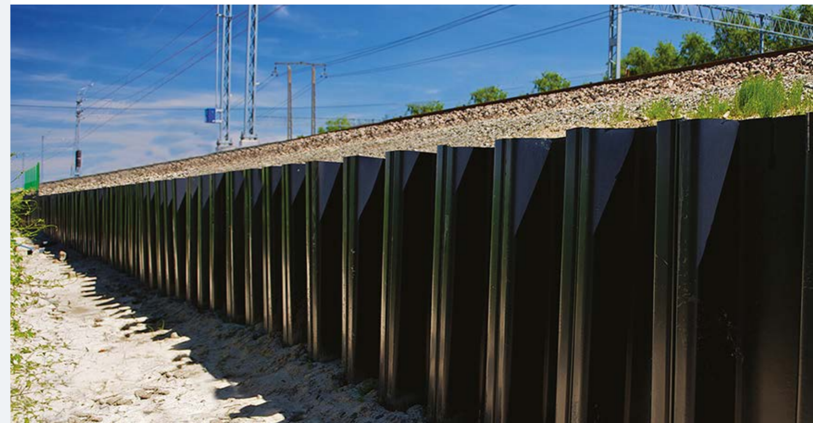
PRUSZKÓW, POLAND: RAILROAD EMBANKMENT STABILIZATION.
