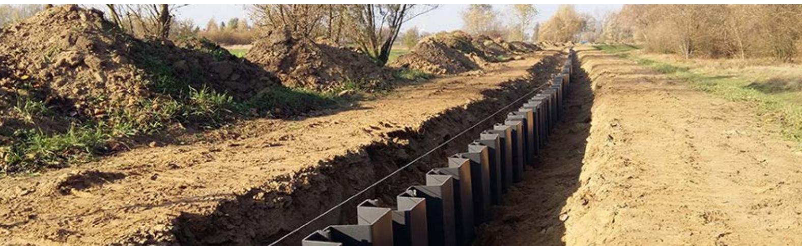
GIZAŁKI, POLAND: REINFORCEMENT OF FLOOD EMBANKMENT.
