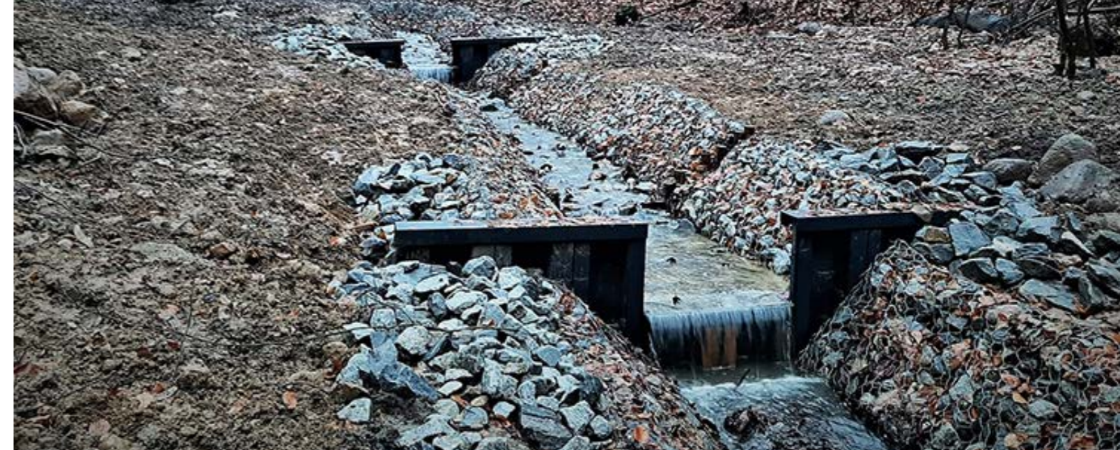
SZCZECIN, POLAND: WATER BARRAGES MADE OF VINYL SHEET PILES FINISHED WITH A CAP.
