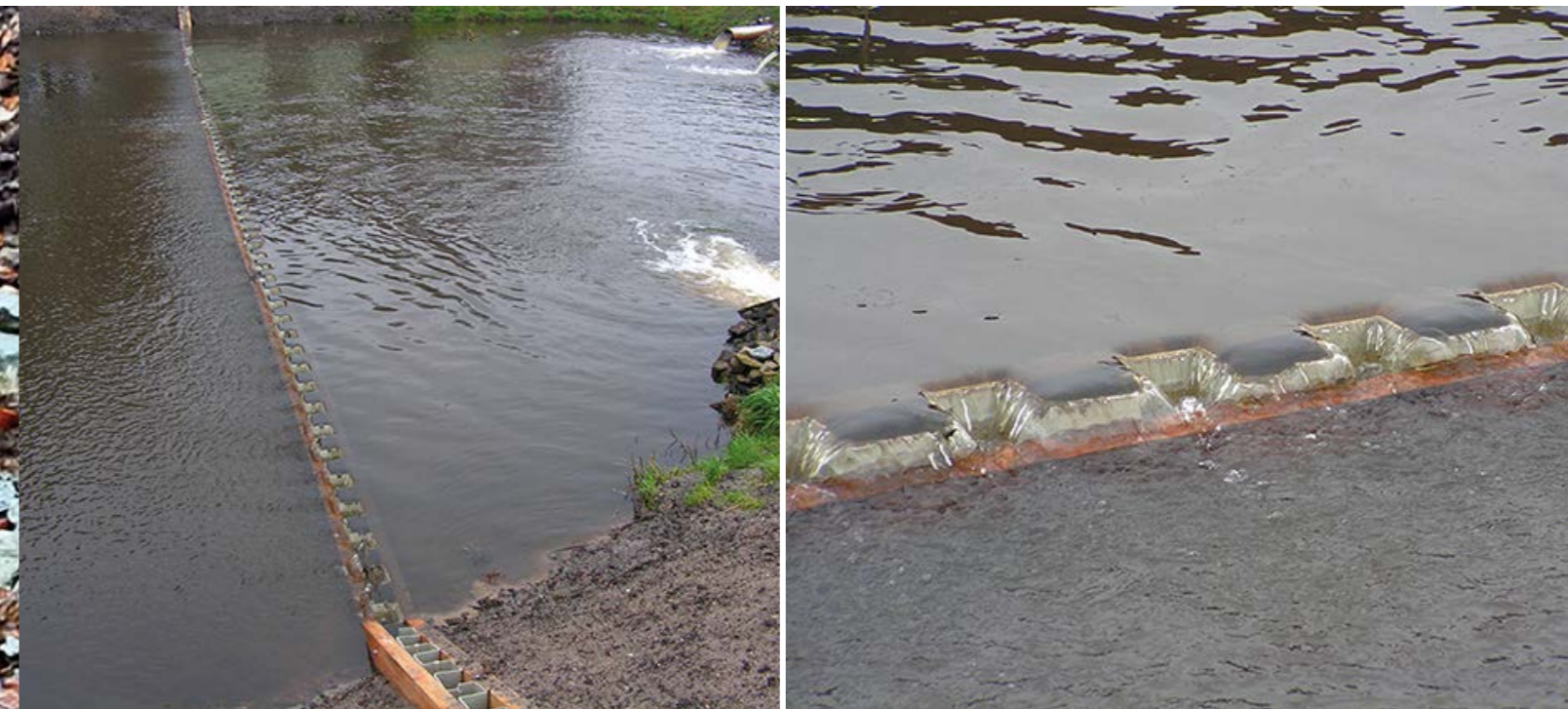
BIESTRZYNNIK, POLAND: ECOLOCK VINYL SHEET PILES USED TO CONSTRUCT A WATER BAR ON THE LIBAWA RIVER IN THE ODER BASIN.
