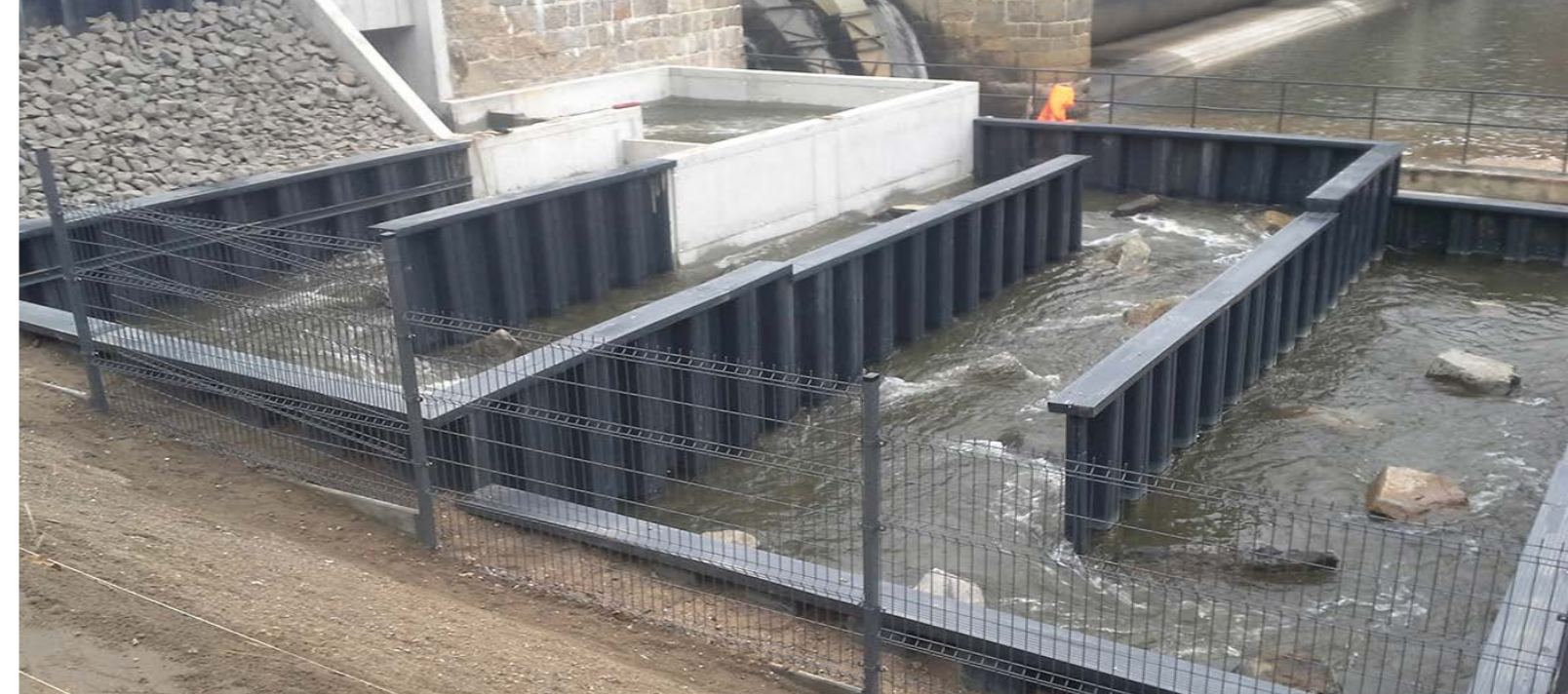
ŻAGAŃ, POLAND: FISH PASS MADE OF VINYL SHEET PILING FINISHED WITH A CAP.
