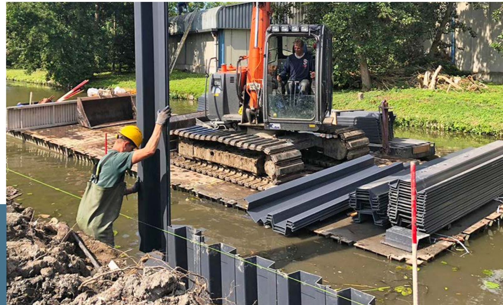
DELFT, THE NETHERLANDS: REINFORCEMENT OF A CANAL EMBANKMENT.
