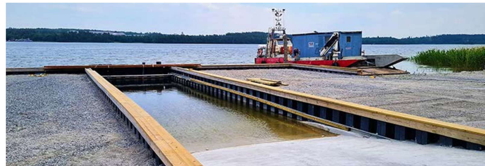
UPPSALA, SWEDEN: HYBRID SHEET PILES USED TO CONSTRUCT A BOAT RAMP.
